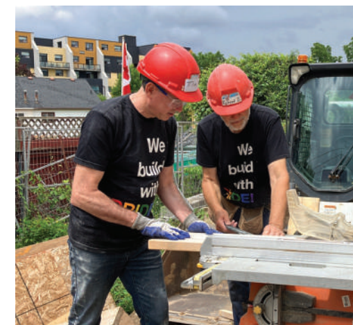
Habitat for Humanity Build - Kitchener
